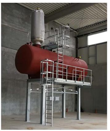
Degasification after erection
