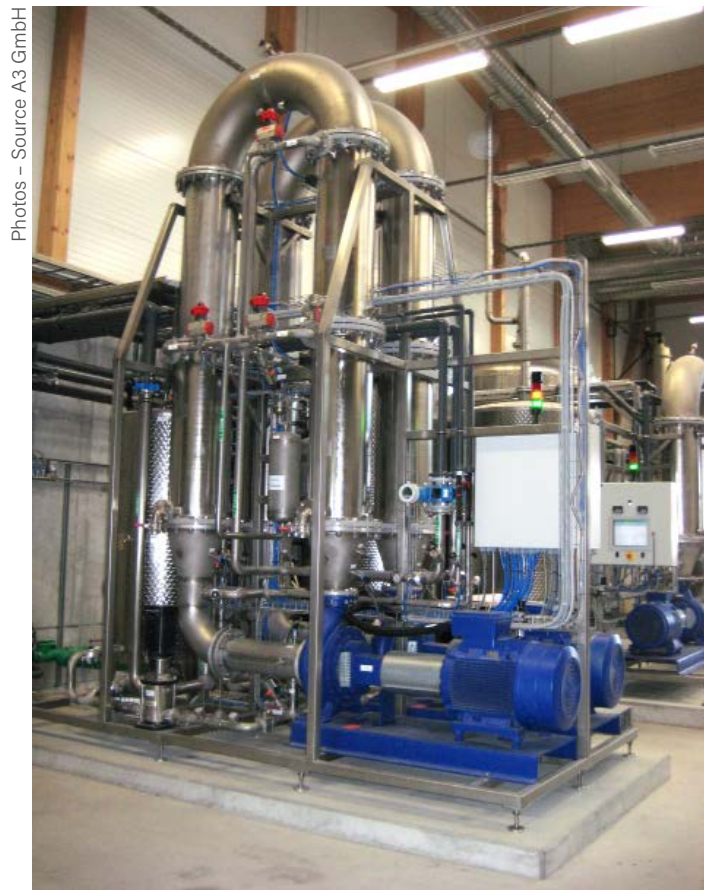
Figure 1: Ultrafiltration with ceramic Multibore tubular membranes
